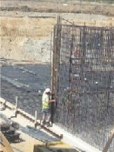
5.5m deep reinforced concrete basement with underground tanks
