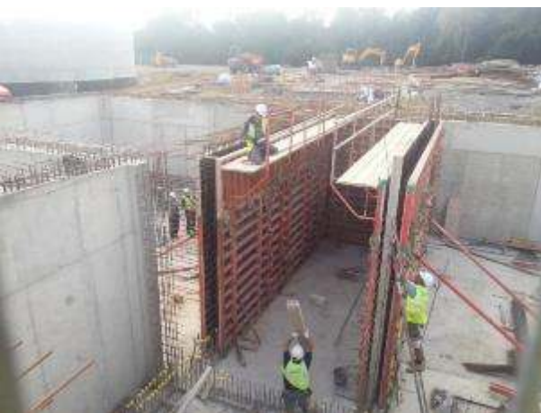
1500m 2 silage clamp with RC retaining walls
