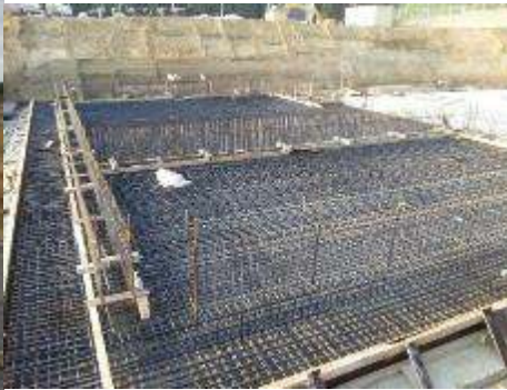
5.5m deep reinforced concrete basement with underground tanks
